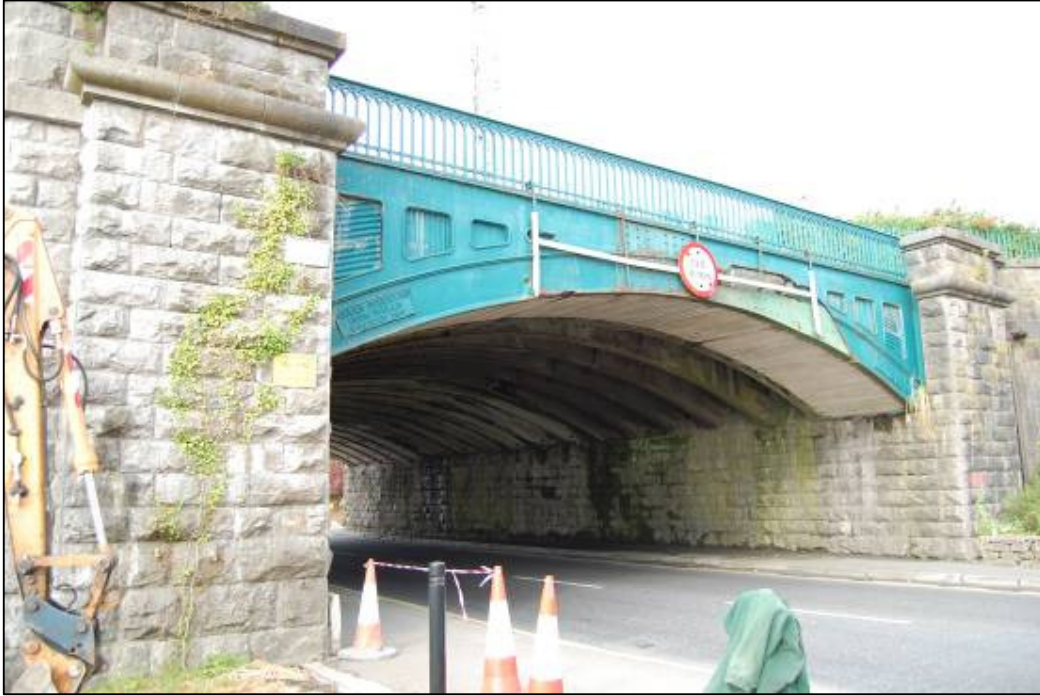
Plate 4 Underbridge (UBG170), from north east.
