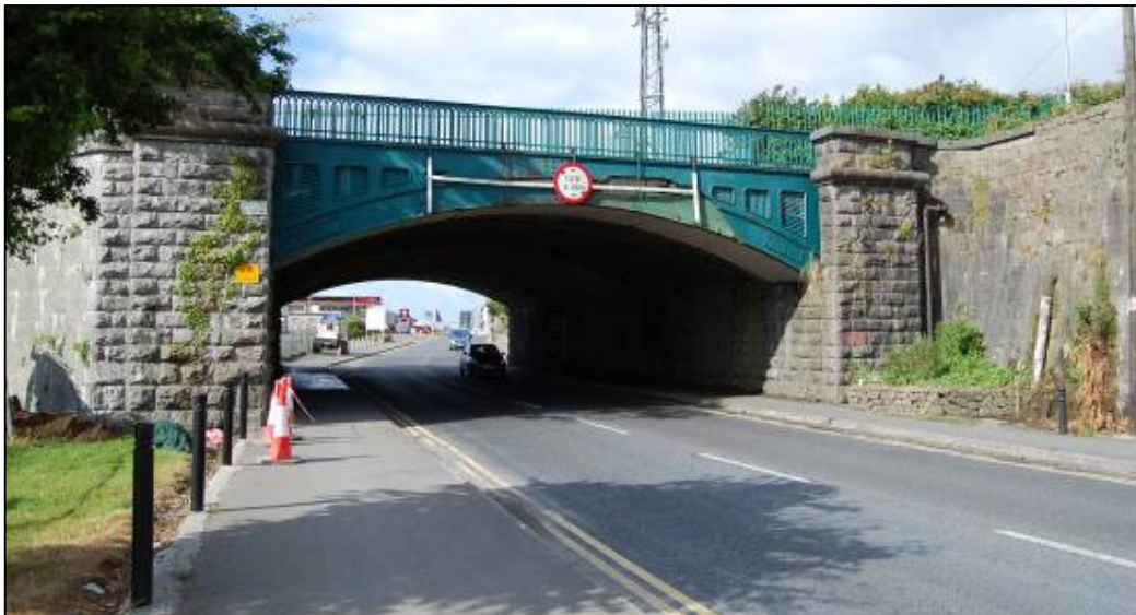
Plate 1 Underbridge (UBG170), from north east.
