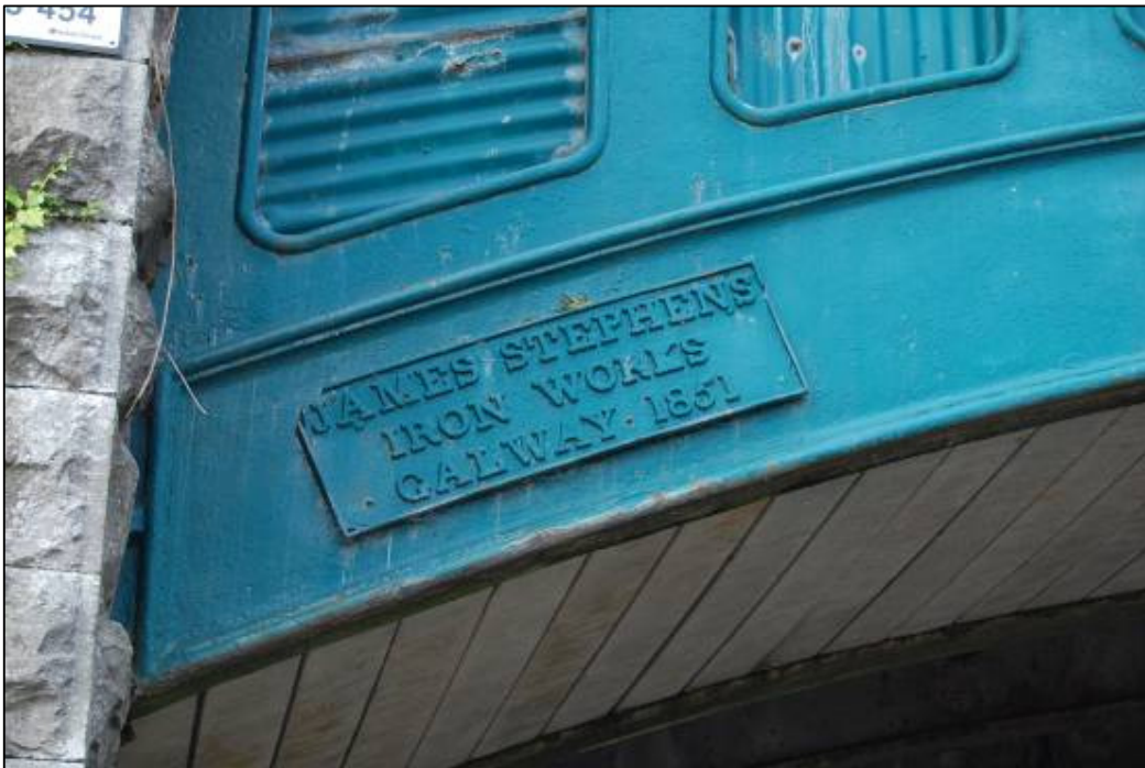
Plate 5 Detail of plate to north east side, 'James Stephens Iron Works Galway 1851'.
