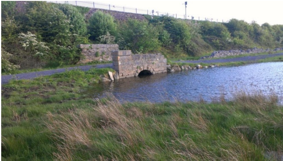
Photo 2 Railway Culvert downstream Face in Lough Atalia at Highwater
