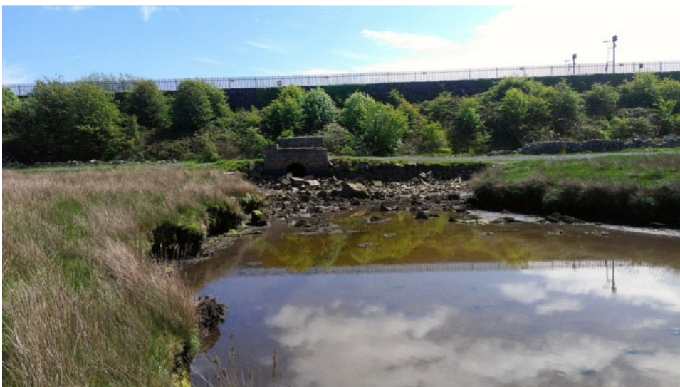
Photo 1 Railway Culvert downstream Face in Lough Atalia at Low-Water
