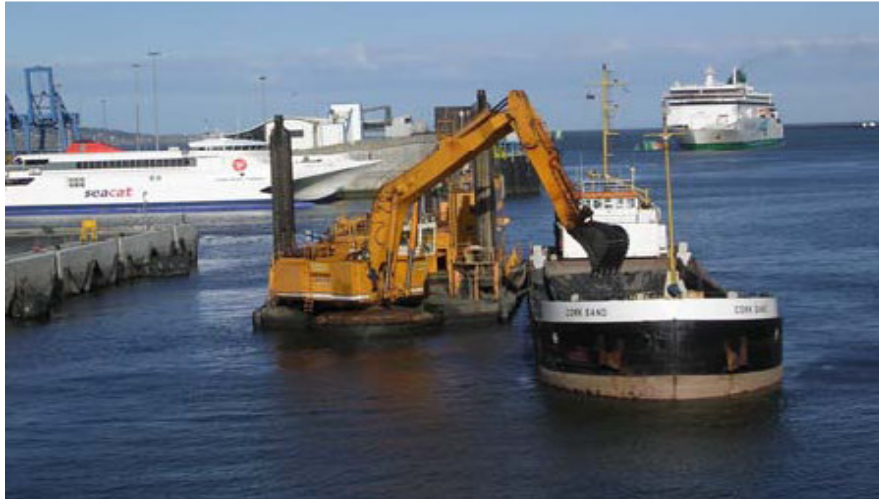
Figure 4.5.11 - Backhoe Dredger loading to a barge
