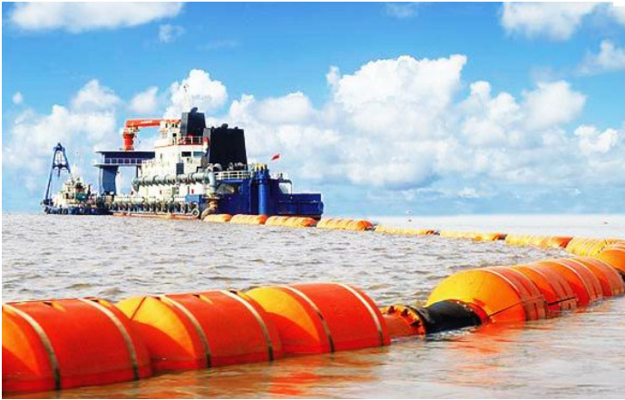
Figure 4.5.10 - TSHD pumping onshore via floating pipeline
