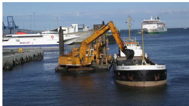
Backhoe Dredger loading to a barge
