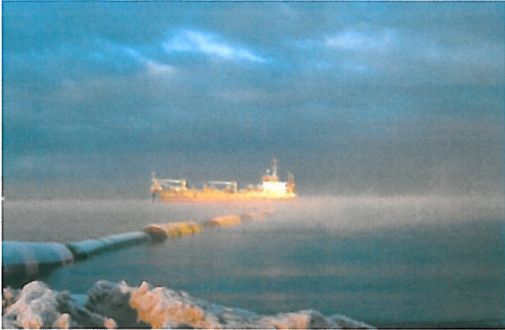
DREDGER TO FLOATING PIPELINE
