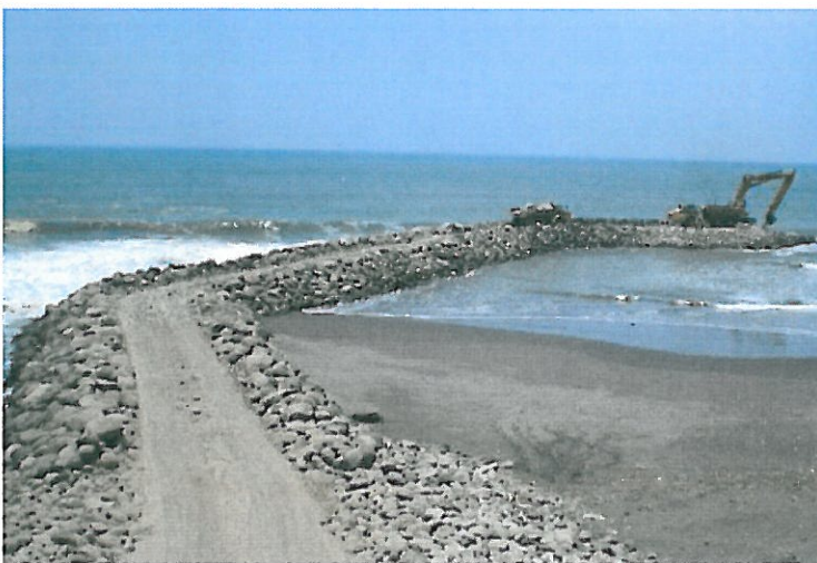
REVETMENT WALL CONSTRUCTION
