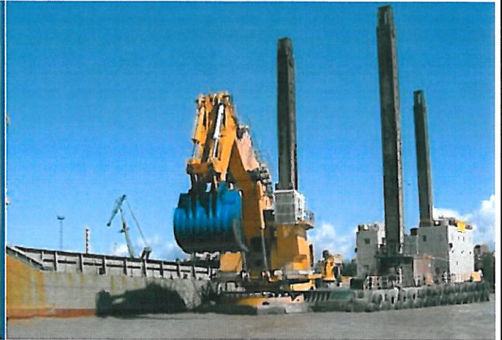
BACKHOE TO BARGE
