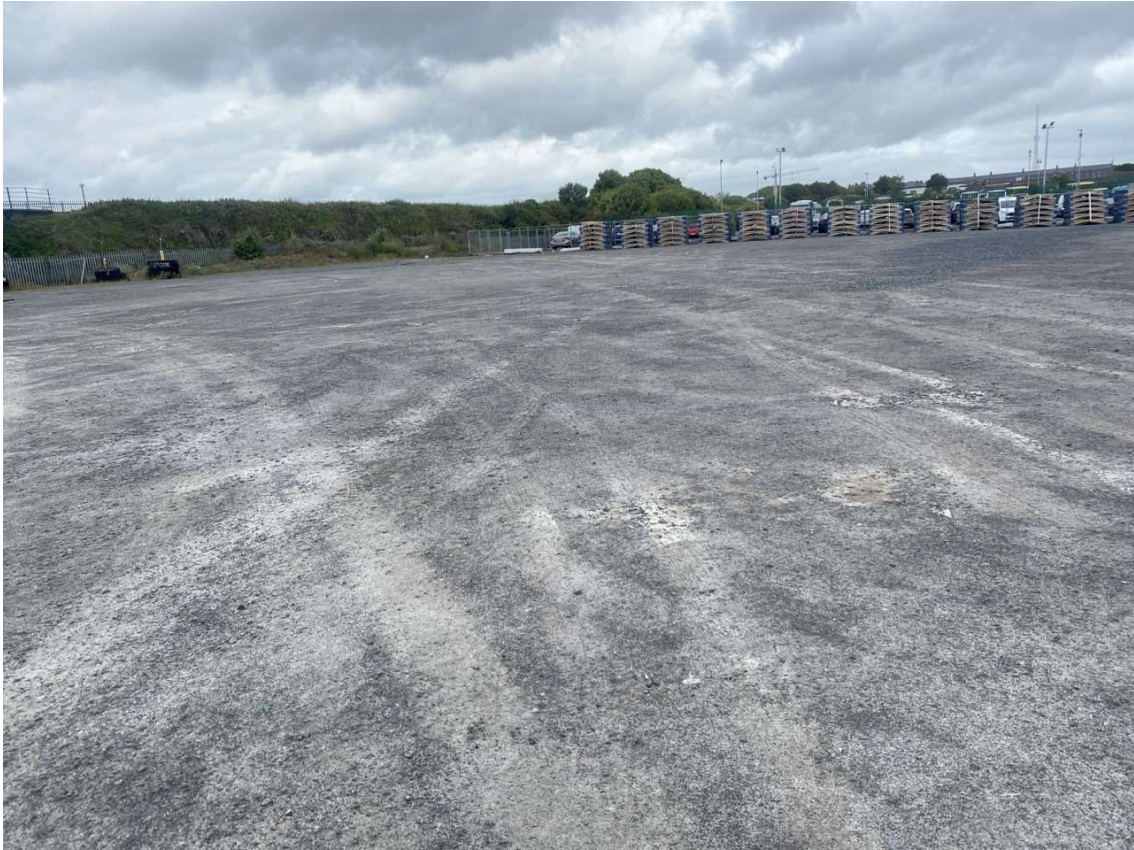
Figure 7-1: Buildings and Artificial Surfaces (BL3) recorded within the proposed development boundary.
