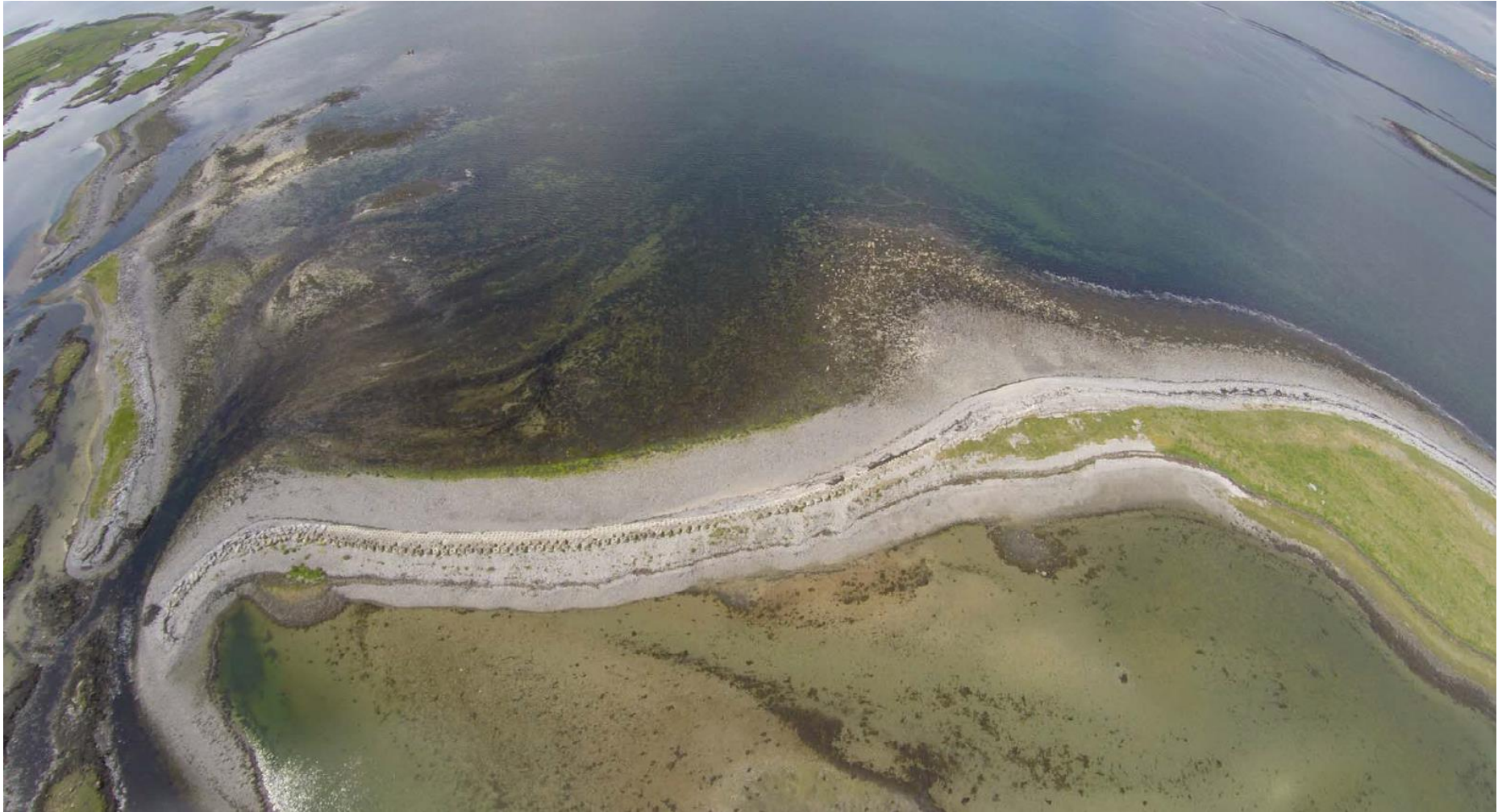
Plate 3. Drone Photo (flown in 2017) of coastal defences and shallow sand intertidal lagoon area behind defences at Lurgan Island
