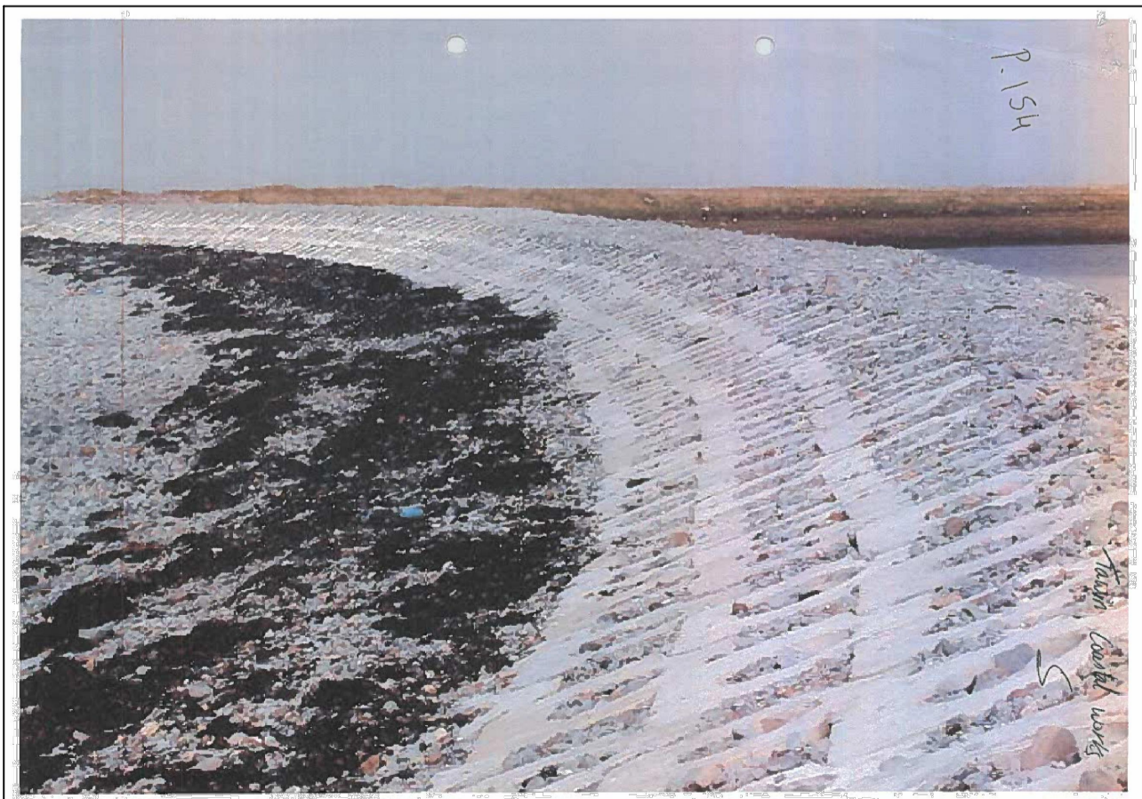
1. Photo at construction
