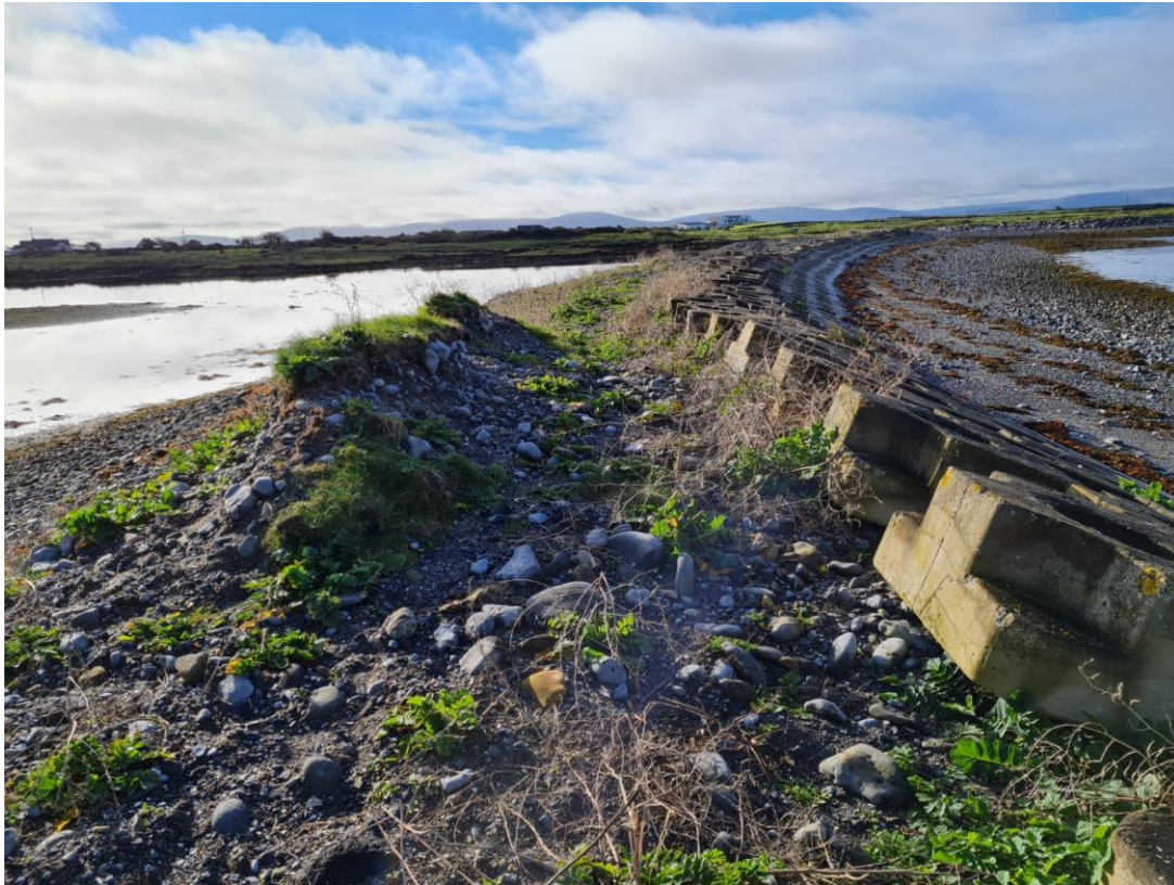
Figure 7-3: Destabilisation of sea defence blocks, Lurgan Island, October 2021.
