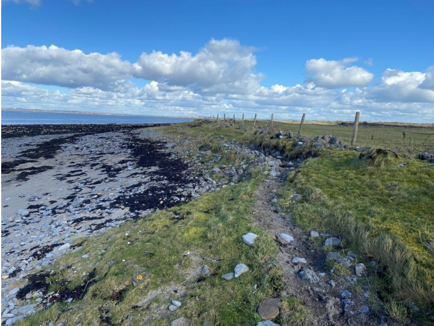
Plate 5. Local Site of erosion on stony bank at subject lands.
