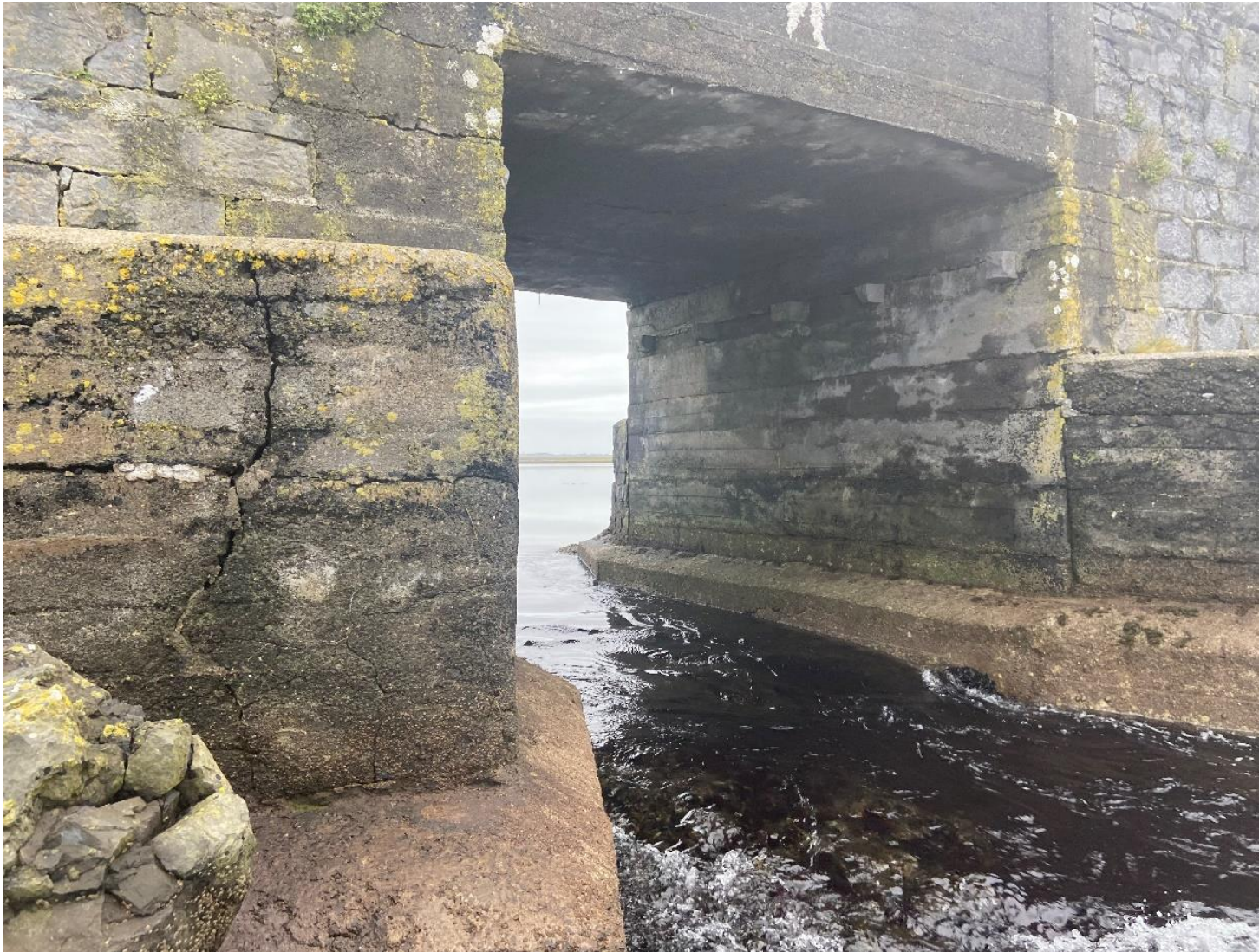
Plate 6 Southern Channel at Ballynacloghy bridge on the Tawin Island local road.
