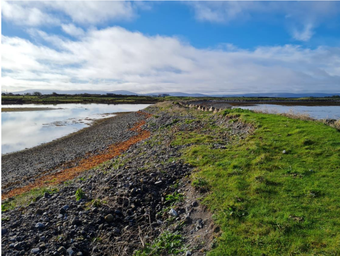
Figure 7-2: Erosion behind sea defence blocks, Lurgan Island, October 2021.
