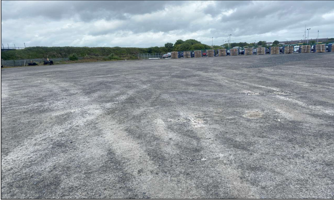
Plate 1 Buildings and Artificial Surfaces (BL3) recorded within the proposed development boundary
